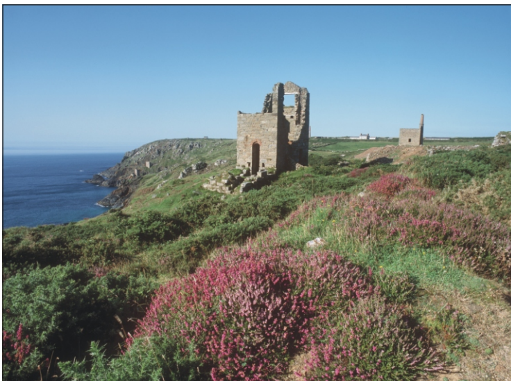
Tin Mine engine house remains, Cornwall AONB. Many protected landscapes in the UK contain sites important for biodiversity conservation, as well as for protection of archaeology, historic buildings and other cultural heritage values. Countryside Agency/Paul Glendell
